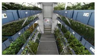
Osram's smart horticulture lighting system prototype used in NASA ground research to help provide space crews with a reliable source of fresh food.
