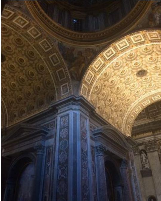
The arc on the left is illuminated by the old lighting system; on the right, the custom-made luminaires from Osram illuminate the arc, clearly highlighting the detail. Picture: Osram
