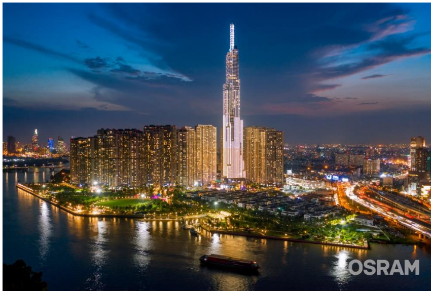
Traxon e:cue provides lighting solutions for Landmark 81, the Highest in Southeast Asia Photo: OSRAM
