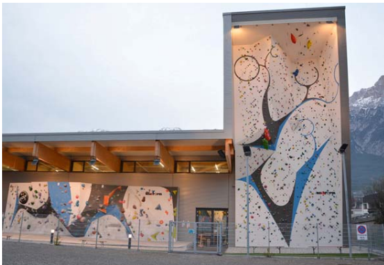
A new paradise for climbers was created in Austria with the "Bergstation" in Telfs.
