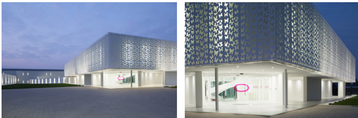
A swarm of backlit butterflies lightly decorates the facade, attracting a high level of attention.
