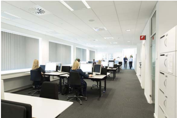
Downlights and louvre luminaires in the offices and conference rooms provide pleasant, VDU-compliant lighting.
